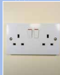
217 electrical systems rewiring
