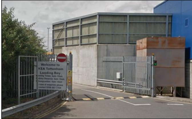
Figure 4 - Existing access to the service yard
