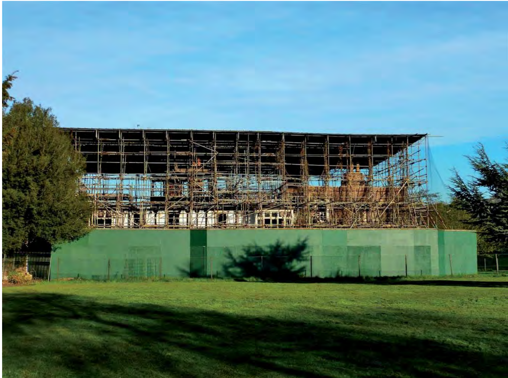
Plate 1: The present exterior of Broomfield House.
