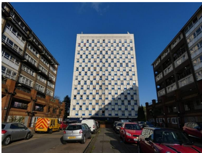
Figure 5 - One of the vacant Shire blocks.
