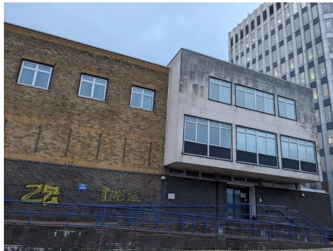
Figure 1 - Vacant police building Enfield Town
