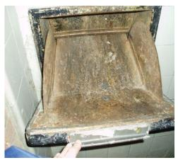
At least one hopper head within the block is blocked with rubbish. There may also be evidence of rotting food and/or maggots within the hopper head.
