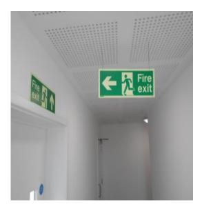
Text: Clear text is often included in fire signs. The text should specify "EXIT," "FIRE EXIT," or other directions like "FIRE ESCAPE," "EVACUATION ROUTE," or "EMERGENCY EXIT."
