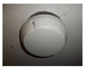
There is clearly a build-up of dirt and cobwebs inside and outside of the light fittings. The cleaning of the light fittings has been neglected and it may have cracks in the surround.
