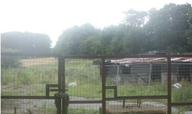
7. Existing gated access to the abandoned stables.
