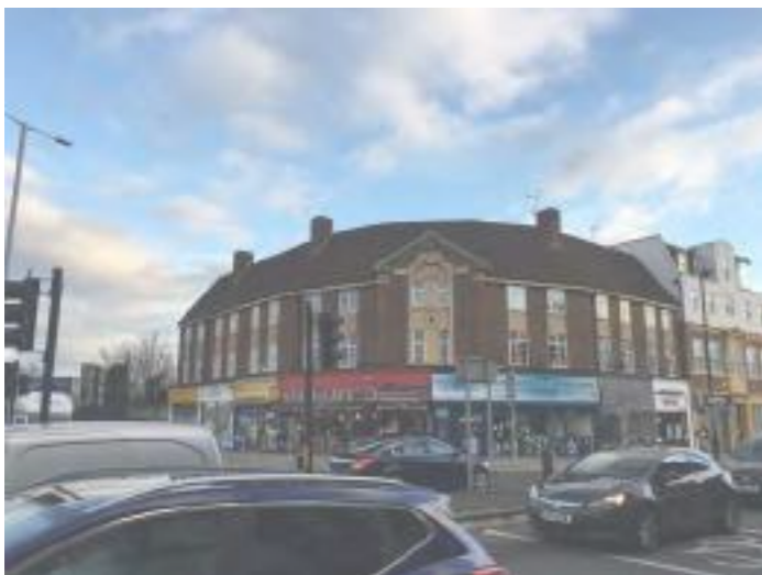
07 / Building opposite site C on Sidney Avenue
