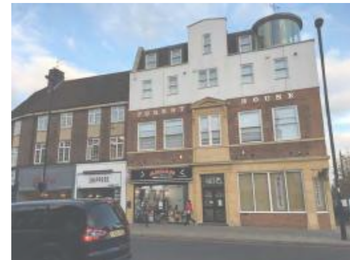
06 / Building opposite Green Lanes terrace
