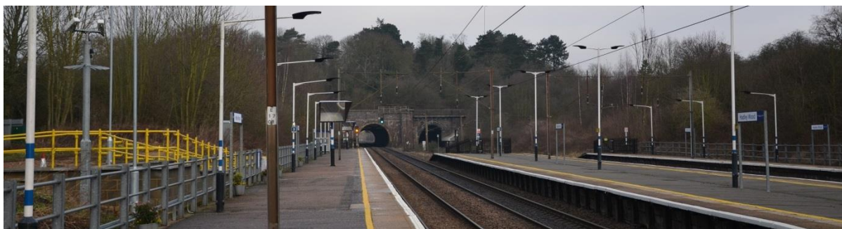
A view from the northbound platform of Hadley Wood Station
