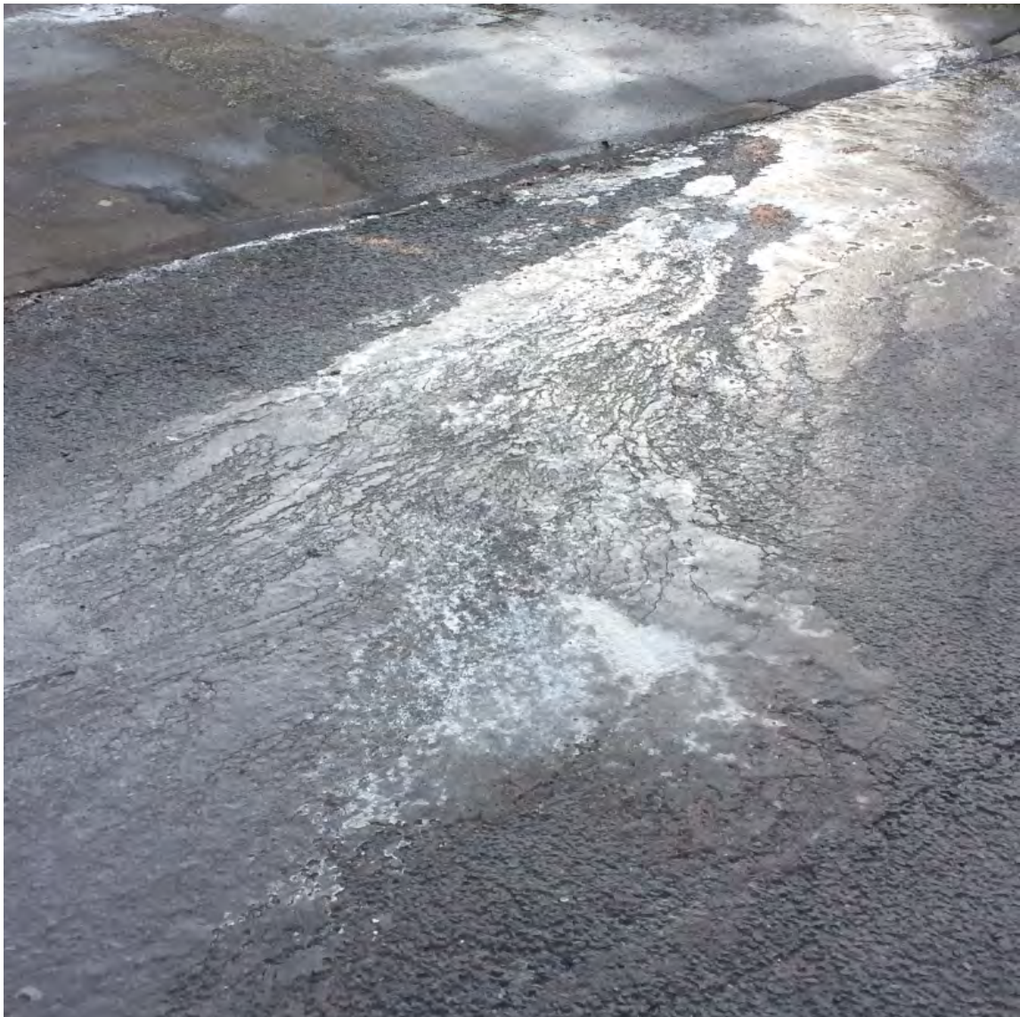
Figure 15: Poor drainage associated with increasing areas of hardstanding have increased occurrences of surface water flooding in Hadley Wood and, as in this example, led to ice on the road in cold conditions
