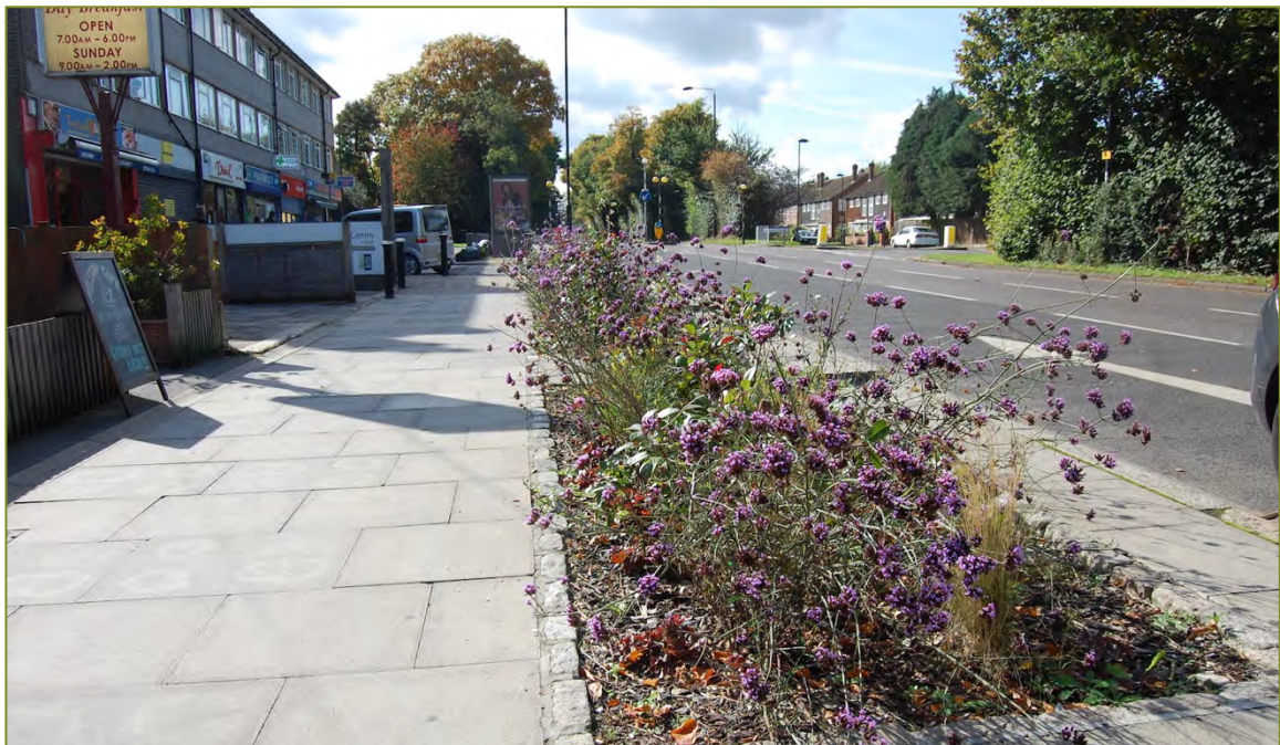
Figure 20: Example of rainwater gardens implemented in Oakwood, Enfield, forming part of the SuDS network (source: Enfield Council)
